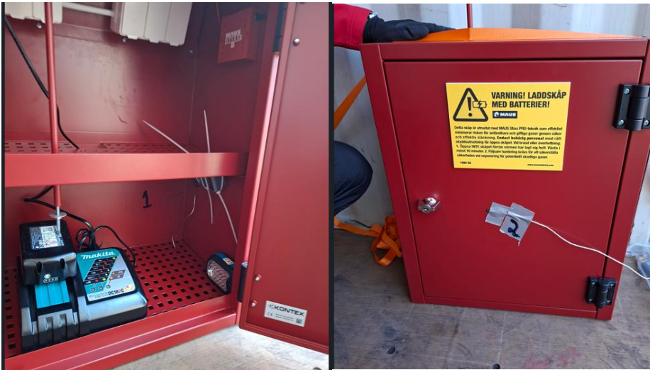
Figure 2 – Configuration of the thermocouples during the test.
